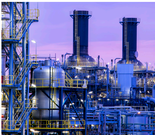
Oil & gas refinery.
